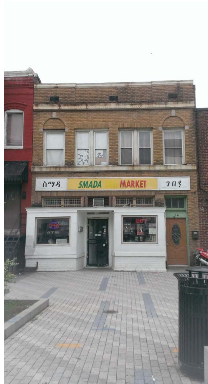
614 T ST, NW LOT 33 TO BE DEMOLISHED
