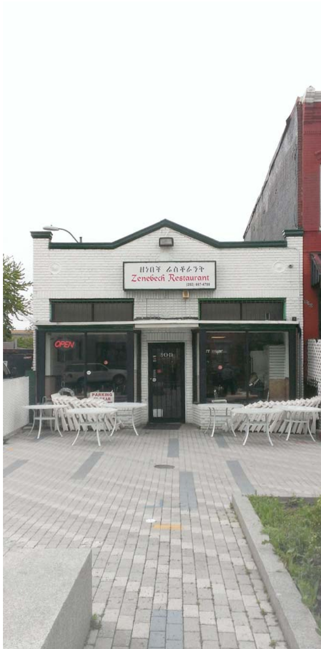
608 T ST, NW LOT 35 TO BE DEMOLISHED
